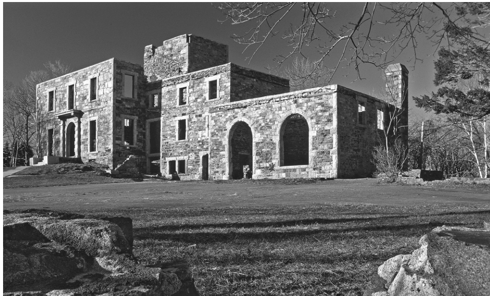
The Goddard Mansion ruins are shown above, with the carriage house on the right, a connector section in the middle and the main part of the mansion on the left.
