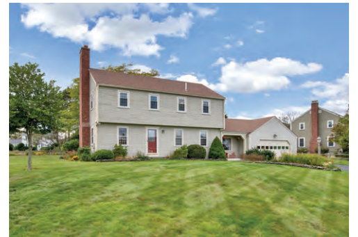
2 ROUNDABOUT LANE LISTED AT $589,000
